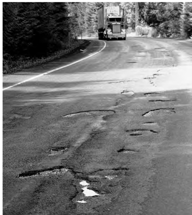
Oregon 58, a major freight route, east of Oakridge shows the signs of surface damage caused by harsh winter weather
