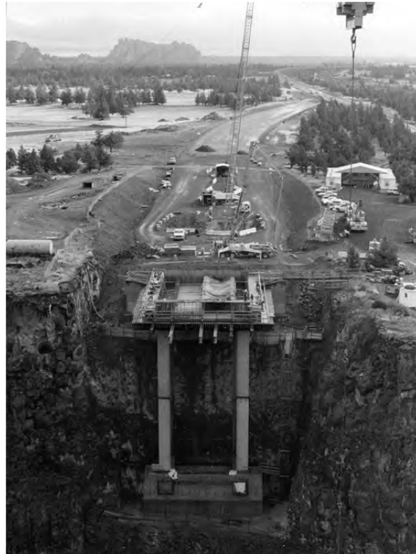
The new Crooked River Gorge Bridge will replace a bridge built in 1924 which cannot carry the increasing traffic on Highway 97.
